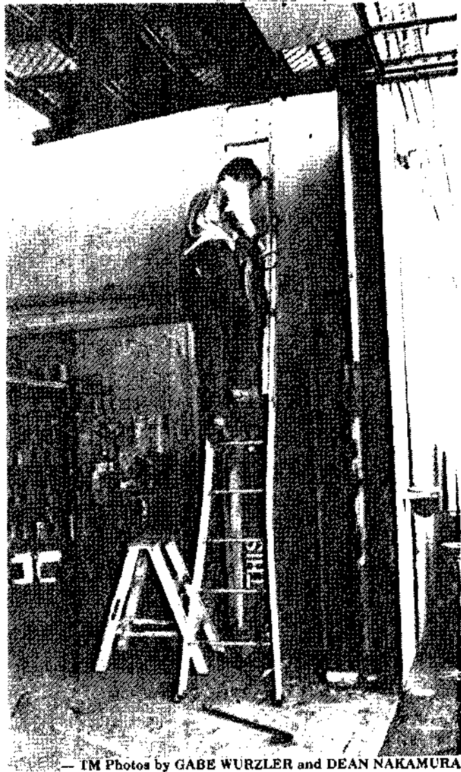
remains pinned after being cut for his release. Top left, door is seen atop paint station wagon. Top right, worker replaces faulty cable that led to the freak accident.
