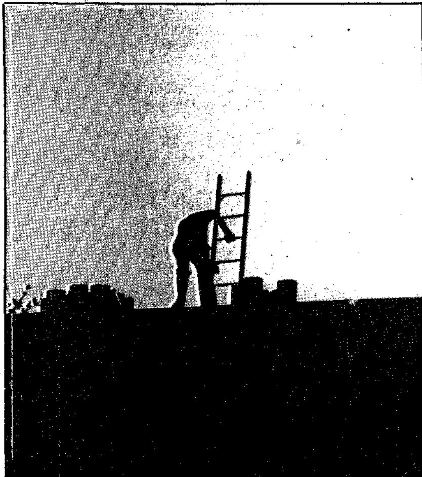
TAR SESSION — Workmen keep busy atop the AC Building being reroofed. TM Photo by B. MICHEL MILBANK
